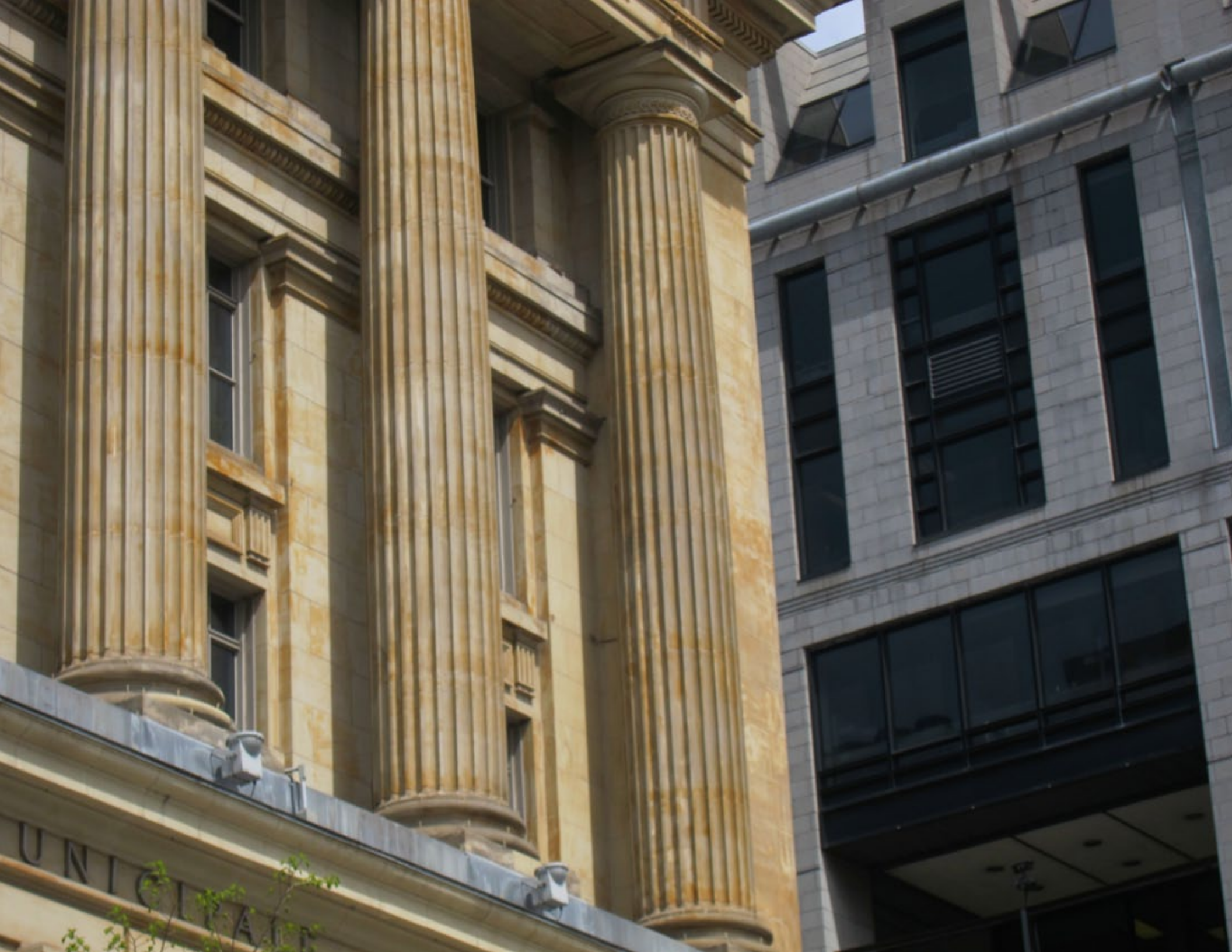
Municipal courthouse & Complexe Chaussegros-de-Léry
